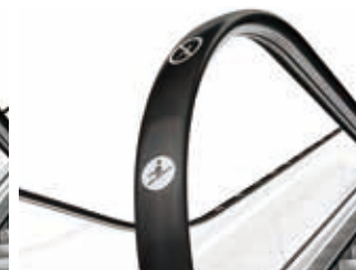
Safety signage handrail
